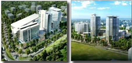
Project: INJ Plaza Location: San Pedro Sula, HN Client: HLARC Status: Design Development
